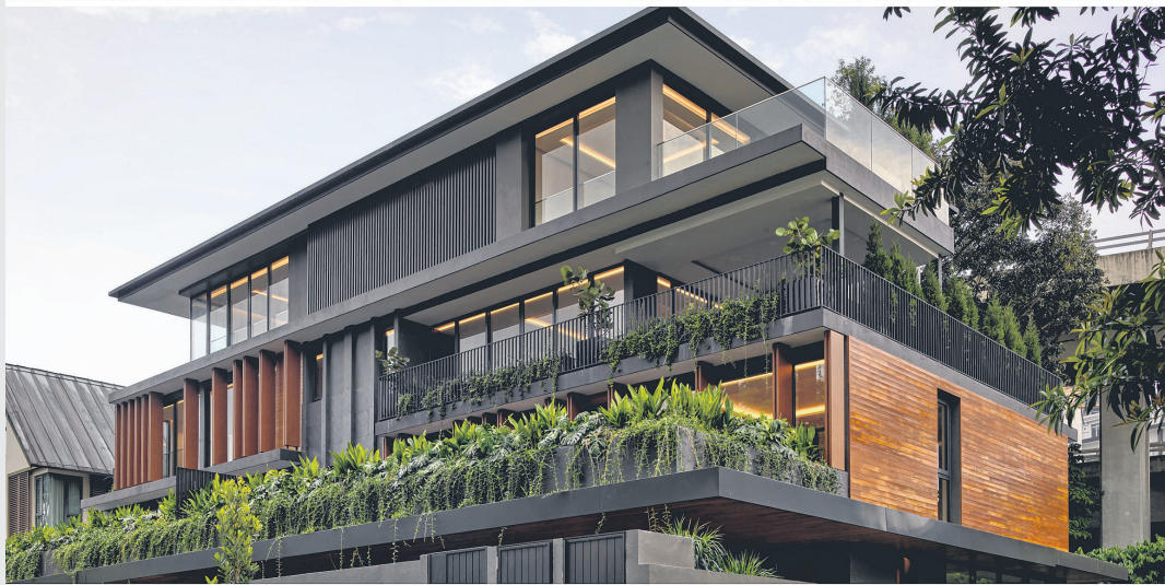
Kapa's pair of semi-detached houses in Westlake Avenue were rebuilt from a bungalow. Rather than produce a mirrored pair, the two homes were designed as a considered whole to look like part of an evolving streetscape. PHOTO: GOOGLE MAPS/KAPA DESIGN CO
